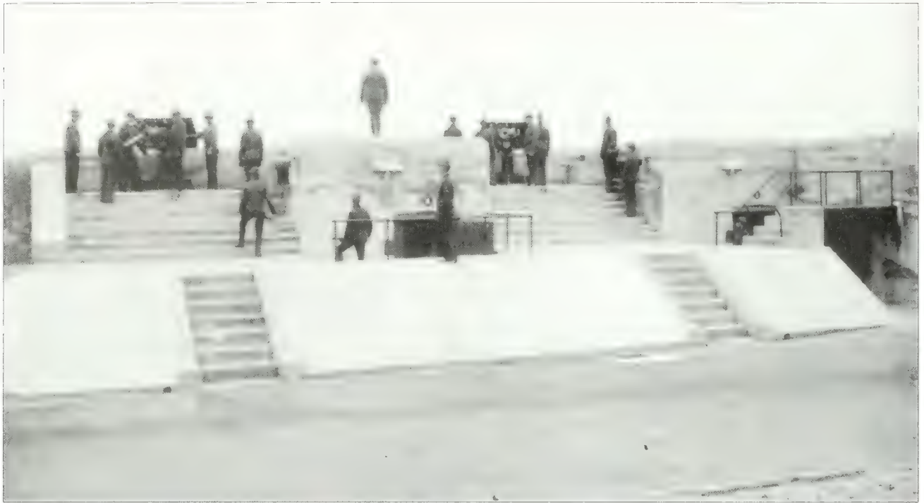
Figure 2.49. View looking northeast at Battery Urmston, circa 1904–08. The commanding officer at Battery Urmston stood on top of the concrete magazine located between two emplacements in order to identify targets and direct the firing of the guns (Thomas Hoffman, Fort Hancock , Charleston, SC: Arcadia Publishing, 2007).
